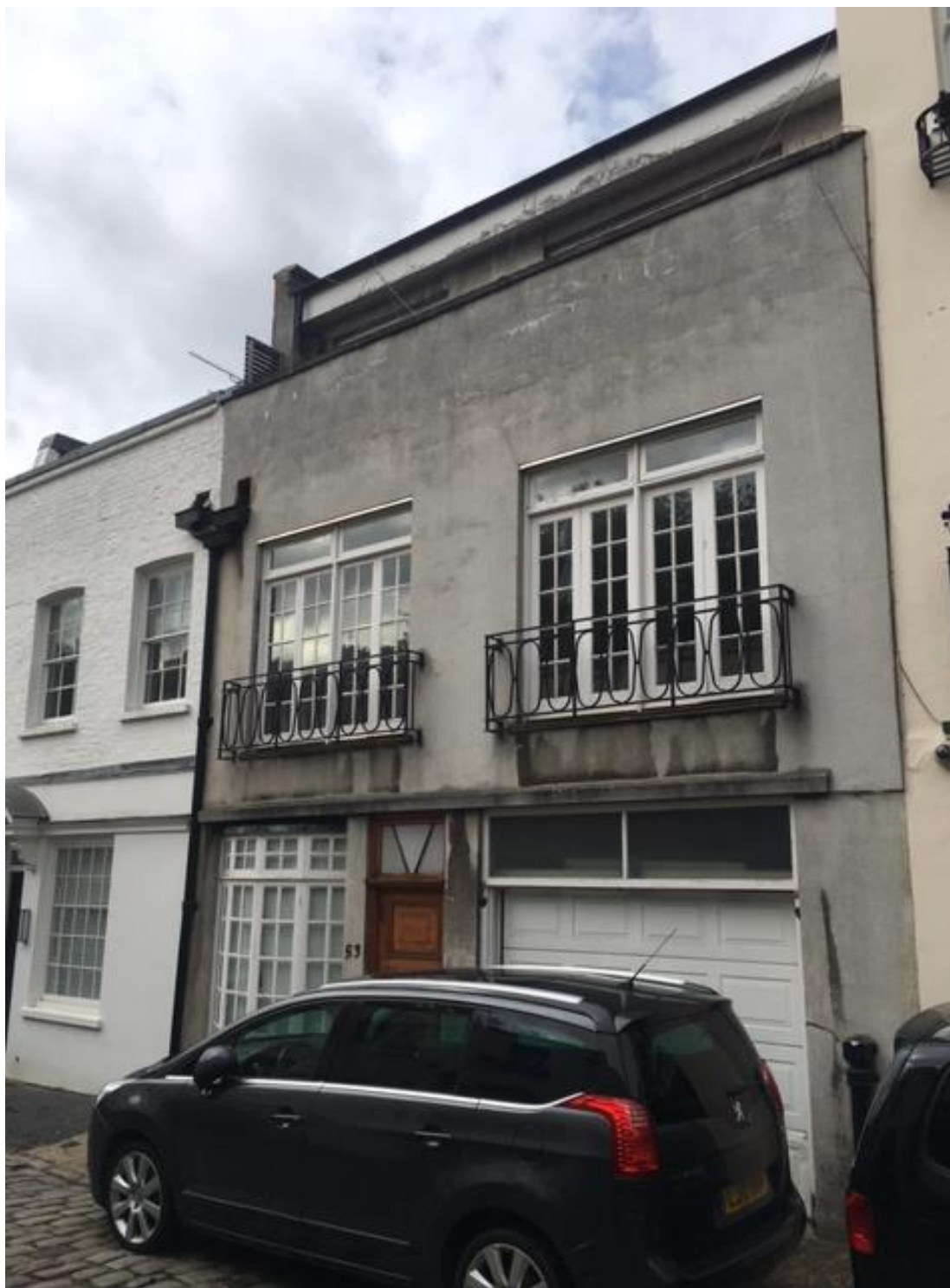
Front Elevation of Application Site
